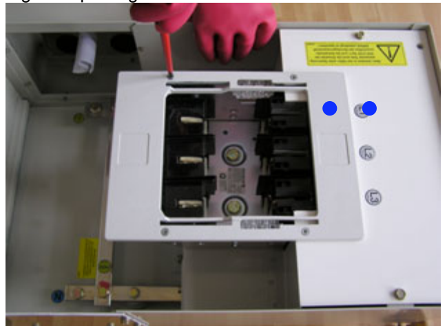
Fig.9: Replacing the fused disconnect switch cover
