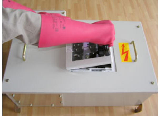
Fig. 4 Opening the fused disconnect switch
