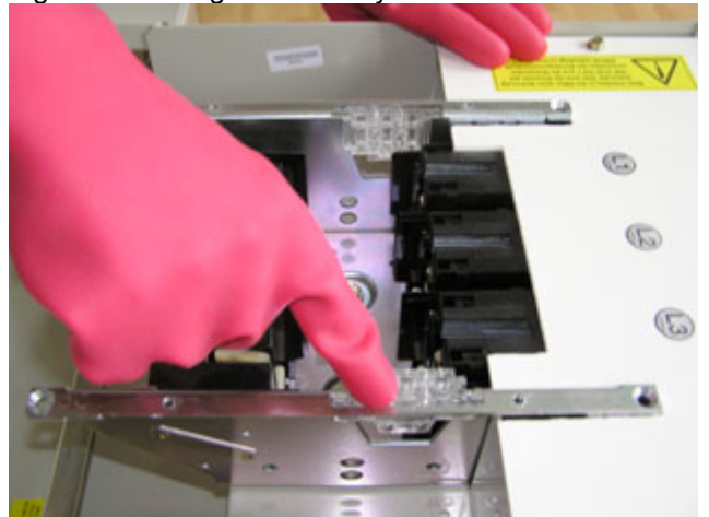
Fig.9: Replacing the fused disconnect switch cover
