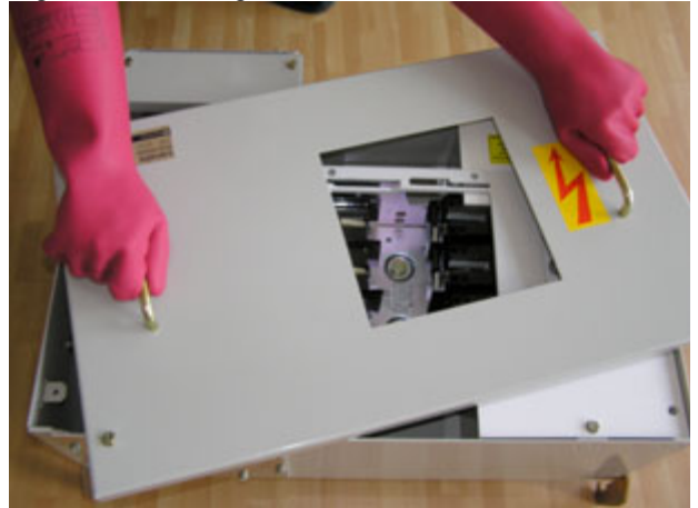
Fig. 7: Marking and removing the cover of the fused disconnect switch
